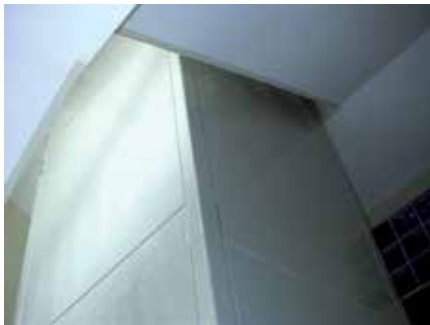
Ill. 4a: Lift shaft with closed sheet steel panels...
